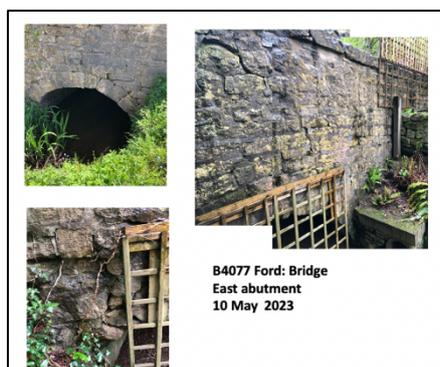
Although vibration recorded was not classed as “significant” the stone arch bridge in Ford, on the B4077, has visible cracks in the east face. This has been reported to GCC Highways. Cracking can be caused by repeated loading, which is possible from the number of HGVs using the B4077.
