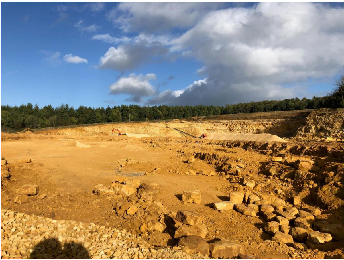
Working face of Oathill quarry looking north and east 20 th October 2021
